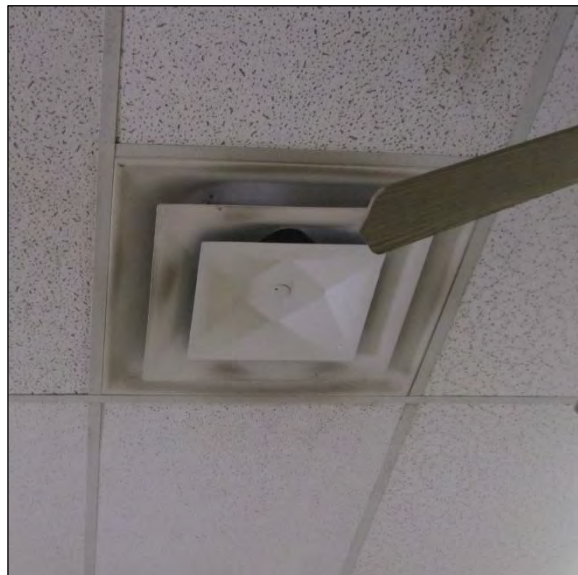
Heavy Dirt in Ventilation System at Fogarty Elementary School
