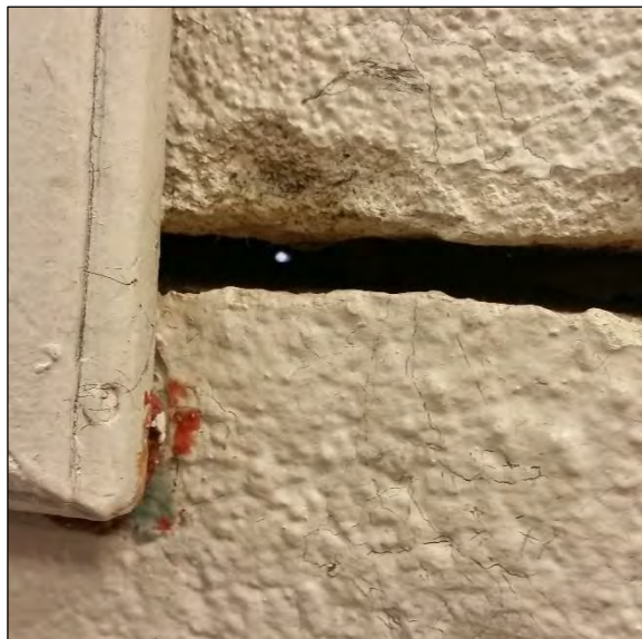
Wall Separation with Daylight Showing in Junior High School
