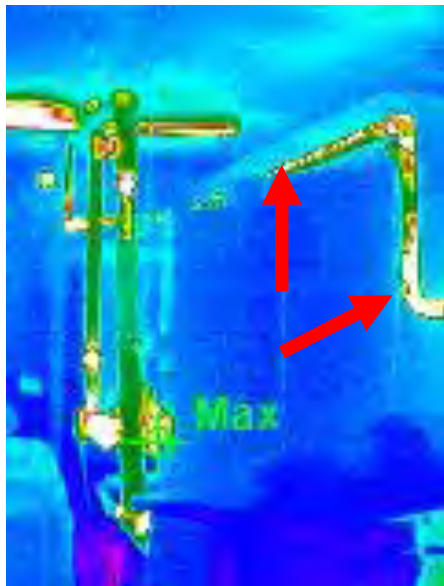
Exhibit 34 GPS – High School – Northwest Mechanical Room Out-going hot water line from water heater should be wrapped in foam insulation
