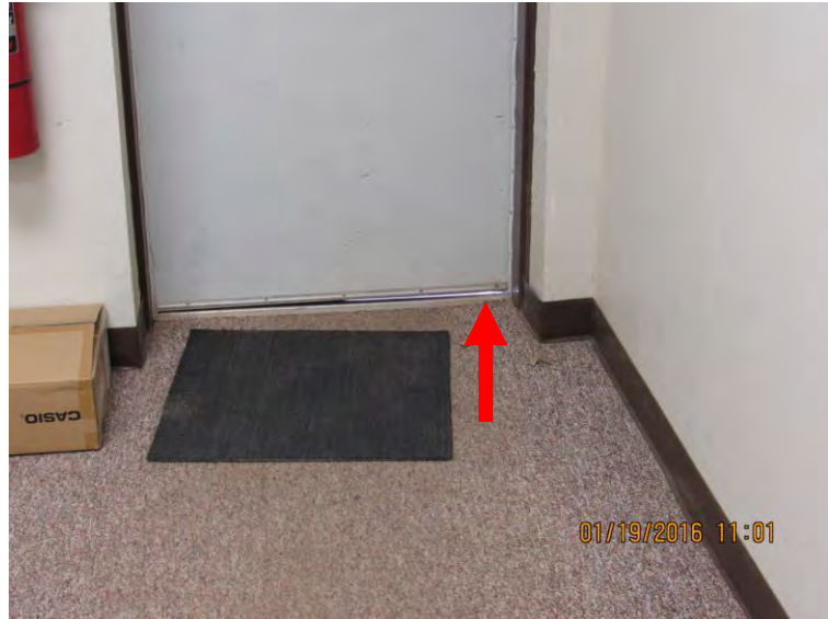
Exhibit 43 GPS – Technology Building – West Entrance Door sweep needs to be replaced
