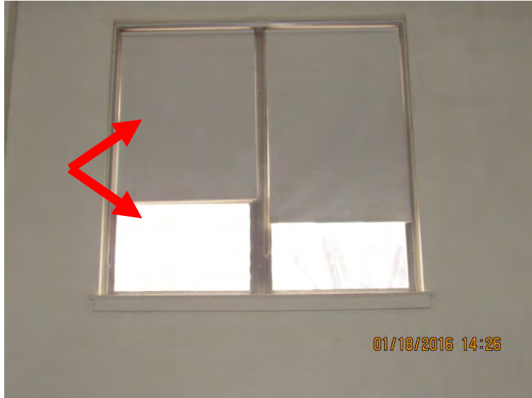
Exhibit 20 GPS – Fogerty Elementary School – Gymnasium Aluminum-framed replacement windows offer little resistance to outside air infiltration but insulated window shades make significant difference compared to just the windows
