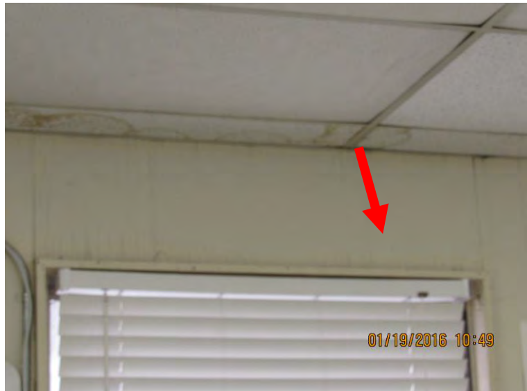
Exhibit 40 GPS – East Transportation Building – Driver's Room Several locations in this room show moisture within the wall from roof leaks
