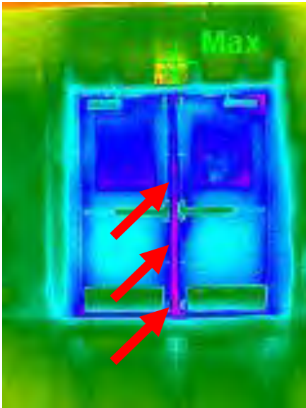
Exhibit 10 GPS – Central Elementary School – West Doors to South Addition Door gasket needs to be replaced
