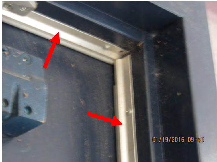
Exhibit 33 GPS – High School – Typical Exterior Door Exterior doors have received weather stripping around their perimeters
