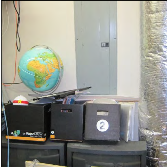
Materials Stored in Front of Electrical Panel in Cottler Elementary School
