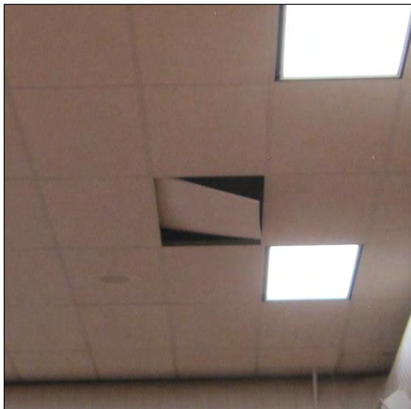
Dislodged Ceiling Tile in Central Elementary Gymnasium
