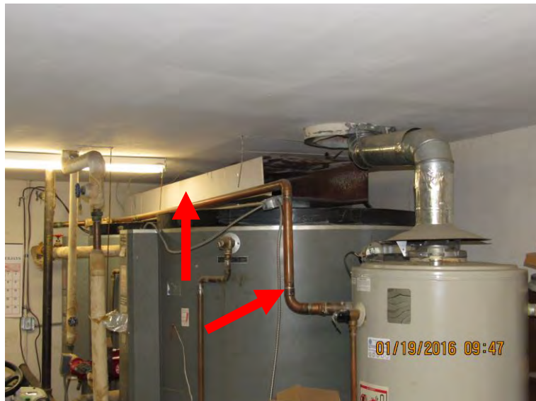
Exhibit 34 GPS – High School – Northwest Mechanical Room Out-going hot water line from water heater should be wrapped in foam insulation
