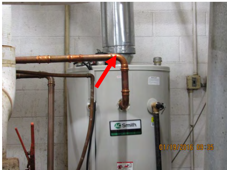
Exhibit 32 GPS – High School – Mechanical Room behind Kitchen (north wall) Out-going hot water line from water heater should be wrapped in foam insulation
