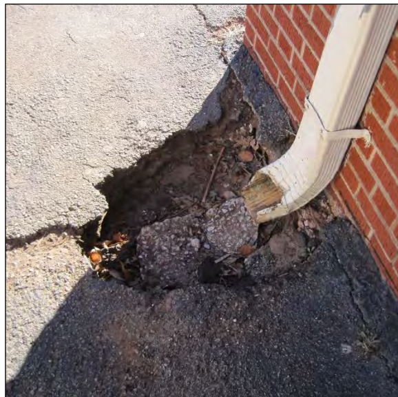
Eroded Asphalt under Down Comer at Cotteral Elementary School
