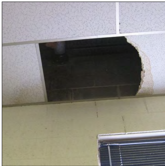
Broken Ceiling Tile in Central Elementary School Kitchen Storeroom
