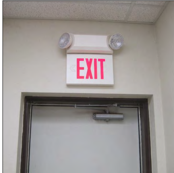
Emergency Combination Light Inoperative in Maintenance Building
