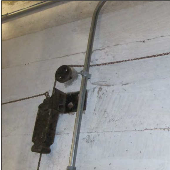
Sliding Fire Door Chain Crimped by Electrical Conduit in Basement of Central Elementary School
