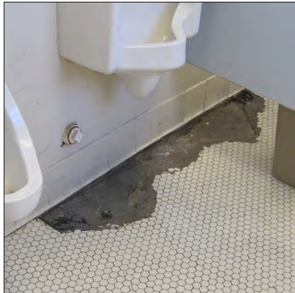
Deteriorated Floor Tile in Bathroom in Junior High School
