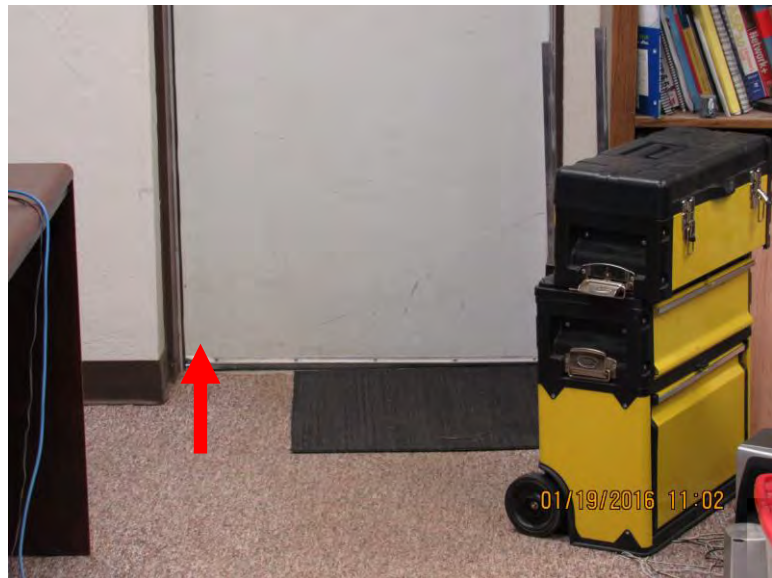
Exhibit 44 GPS – Technology Building – East Entrance Door sweep needs to be replaced
