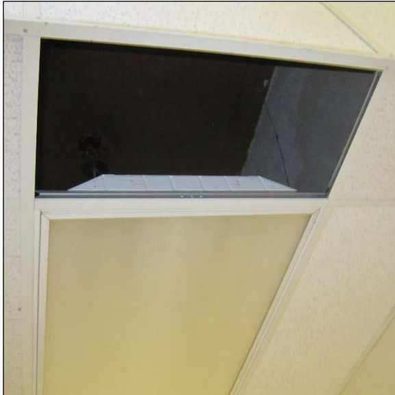
Broken Ceiling Tile in Central Elementary School Kitchen Storeroom
