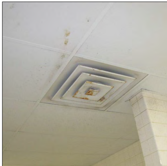
Rust and Stains on Diffuser in Boys Bathroom in High School
