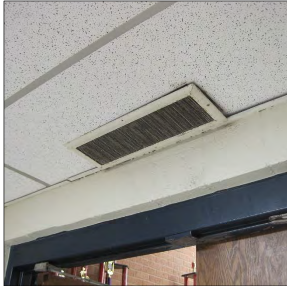
Rust and Stains on Diffuser in Boys Bathroom in High School
