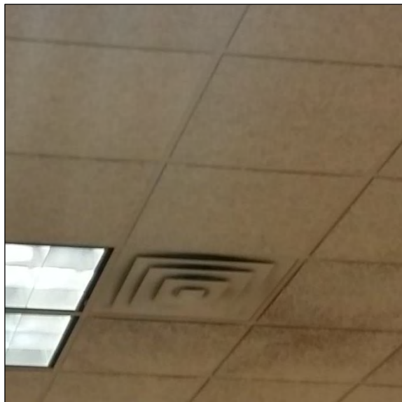
Dirt Pattern Around Diffuser Indicates Vent System Needs Cleaning in GUES
