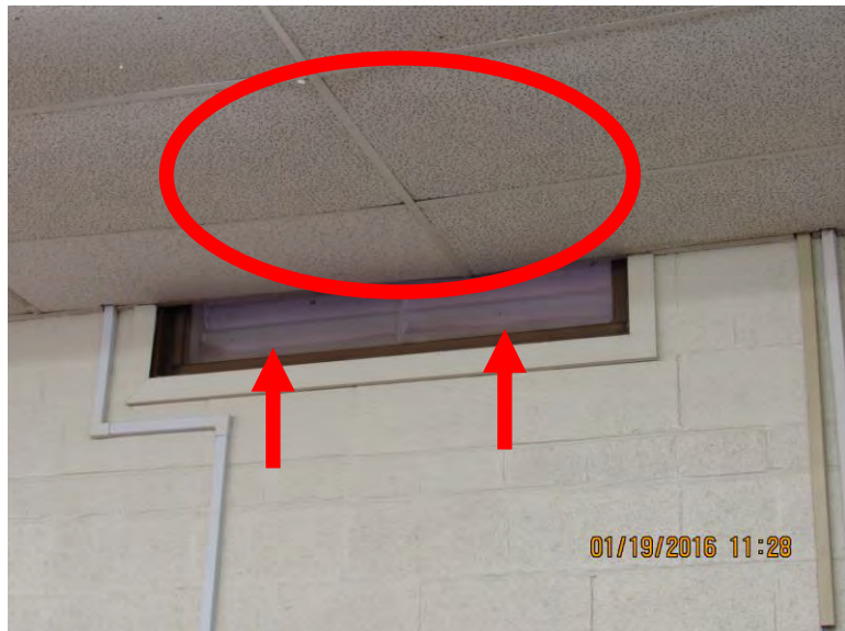
Exhibit 46 GPS – Faver Alternative School – NW Classroom of NW Building Windows hidden behind ceiling tile are allowing outside air and water to infiltrate
