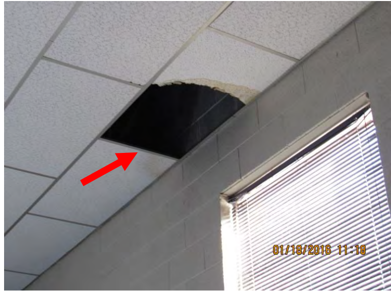
Exhibit 9 GPS – Central Elementary School – Gymnasium Tile ceiling forms a significant barrier to cold air
