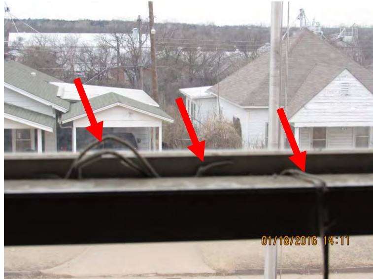
Exhibit 19 GPS – Fogerty Elementary School – Typical Classroom Gasket material has failed and needs to be replaced
