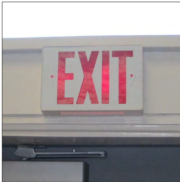
Exit Sign at North Exit from Board Room Cannot be Tested as Installed
