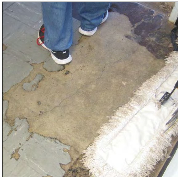
Deteriorated Floor Tile in Cafeteria at Cotteral Elementary School
