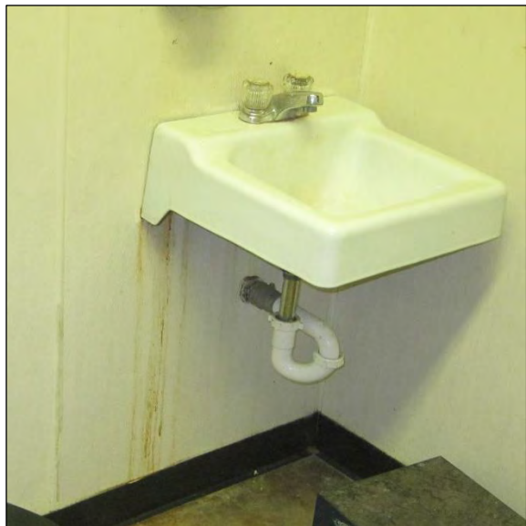
Stained Wall under Lavatory in Portable at Cotteral Elementary School
