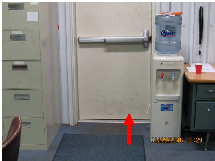
Exhibit 38 GPS – Building of Champions – West Entrance Door sweep needs to be replaced
