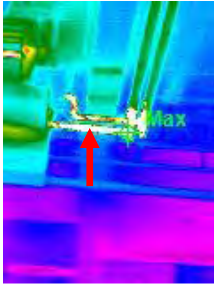
Exhibit 35 GPS – High School – Gymnasium – Typical Air Handling Unit (4) In-coming hot water lines should be wrapped in foam insulation
