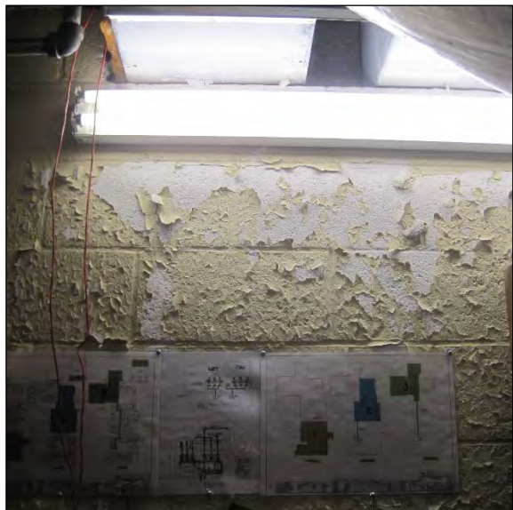
Peeling Paint in Riser Room in High School
