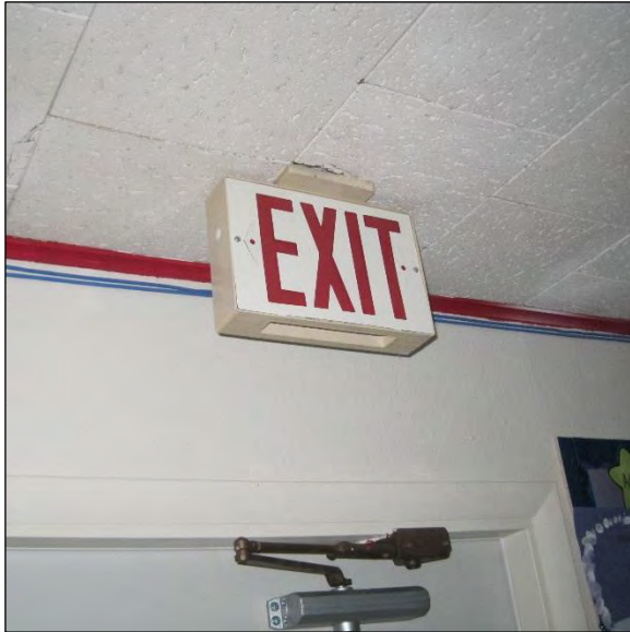
Exit Sign at North Exit from Board Room Cannot be Tested as Installed
