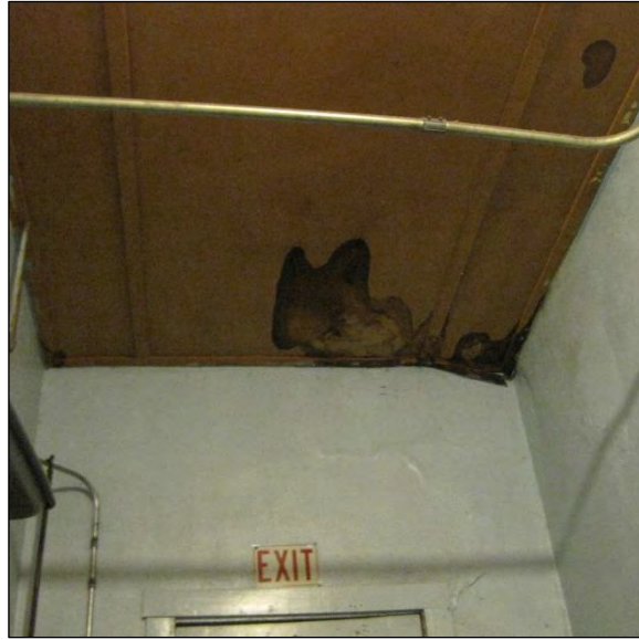
Heavy Dirt in Ventilation System at Fogarty Elementary School
