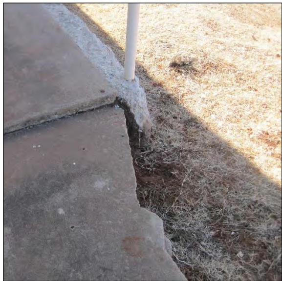
Dangerous Erosion Around Sidewalk Along High School Vo-Ag Building
