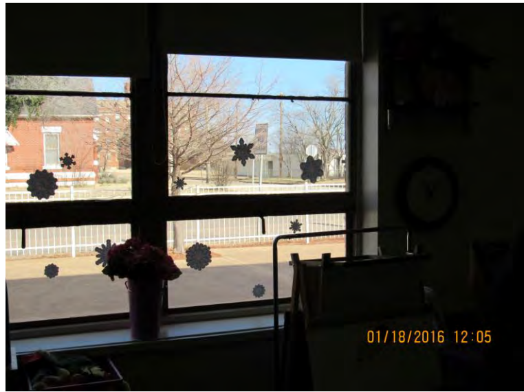
Exhibit 13 GPS – Cottler Elementary School – Typical Classroom Original steel-framed windows offer little resistance to outside air infiltration
