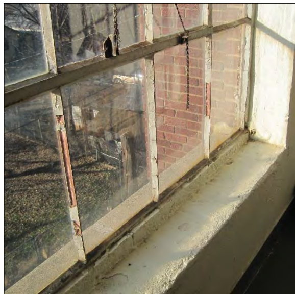
Deteriorated Window Frame on Second Floor in Junior High School
