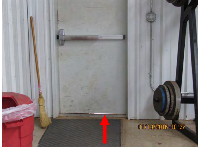
Exhibit 39 GPS – Building of Champions – North Entrance Door sweep needs to be replaced
