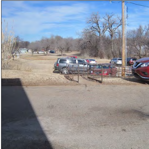
Handicapped Ramp from Junior High School to South Portable Lacks Hand Rails
