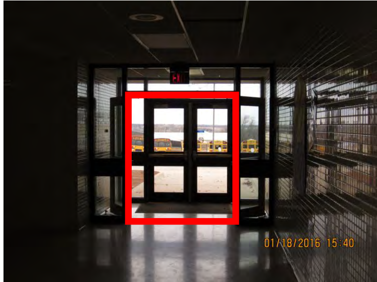
Exhibit 25 GPS – Upper Elementary School – West Entrance Vestibule doors left open is like a 6’x6’ hole in the building exterior
